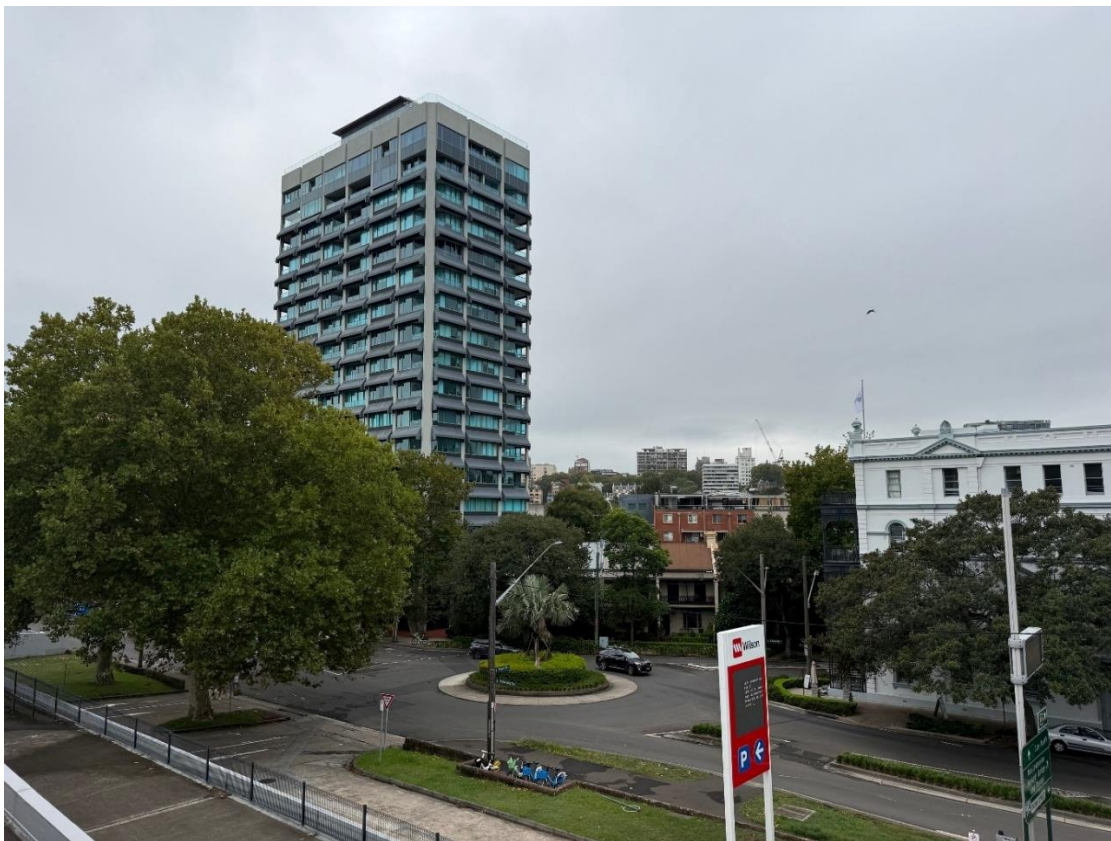
Figure 4: Site viewed from the Domain looking north-east
