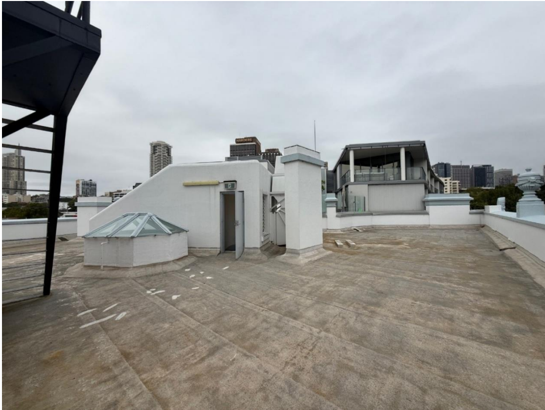
Figure 7: Existing roof top looking south-west
