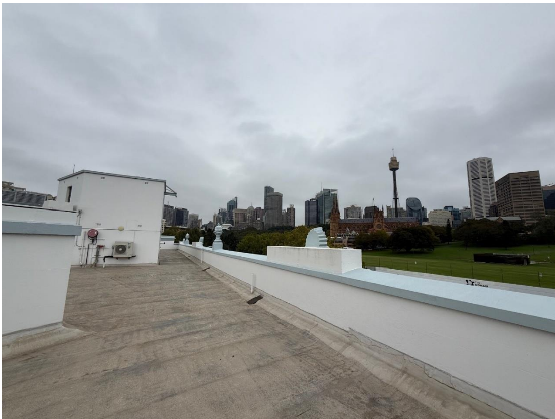
Figure 10: Existing rooftop looking south - west
