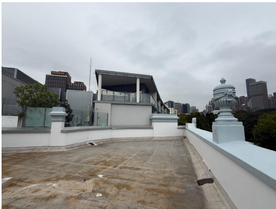
Figure 24: The proposed acoustic screen wall will abut the western parapet immediately adjacent to the decorative urn - existing roof top looking south-west
