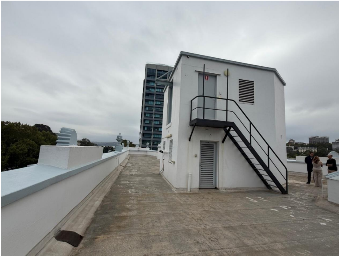
Figure 9: Existing rooftop looking north
